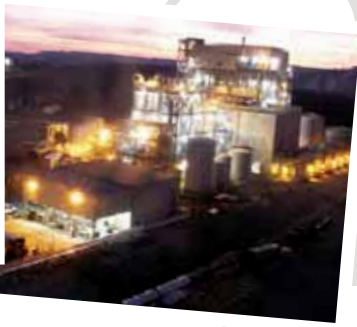
Loudon Bio-PDO™ plant, US, 2004
