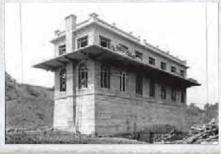
Staley Pump House and Fellowship Club
