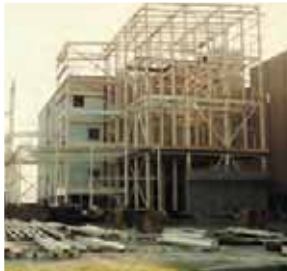
The KRYSTAR® building under construction in the 1980s
